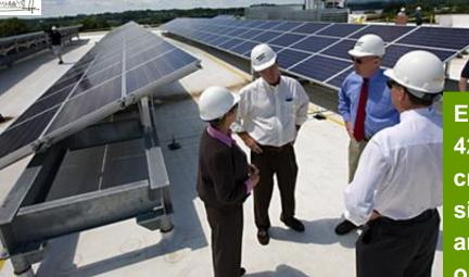
Evergreen Solar 42 kW crystalline silicon solar array, installed on roof of Campus Square Building
