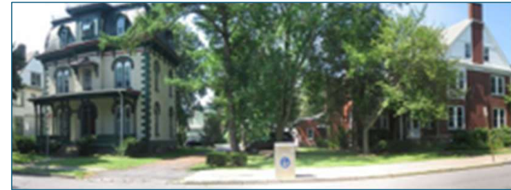
Water Street Historic District, Lock Haven Clinton County Zoning overlay historic district
