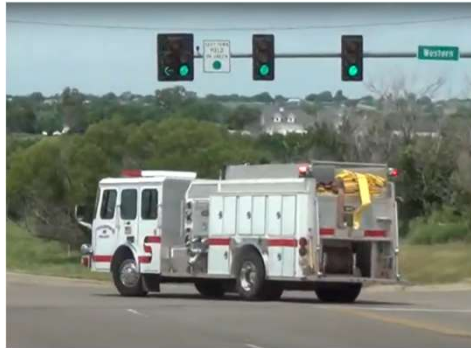
Emergency Services Signal Preemption (With repeater poles to detect around curves)
