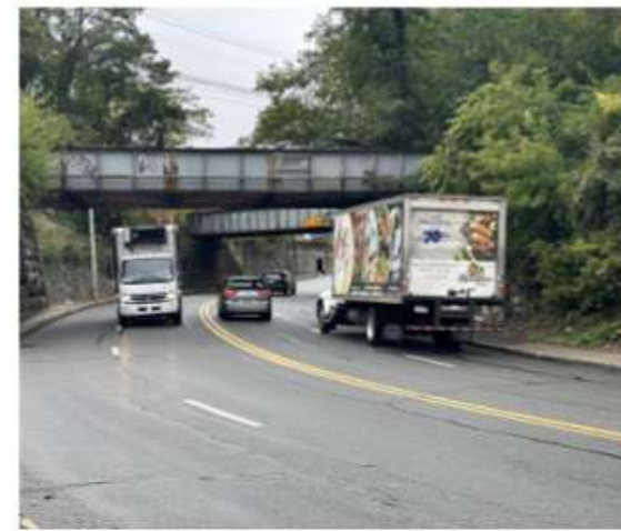
Corridor pinch point with two NS overhead railroad bridges looking westbound
