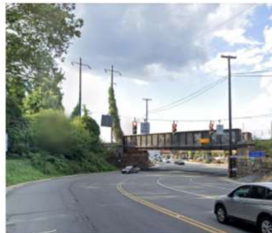
Approaching Front Street intersection looking eastbound
