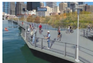
Boardwalk section from Locust Street to South Street currently under construction (Source: SRDC)
