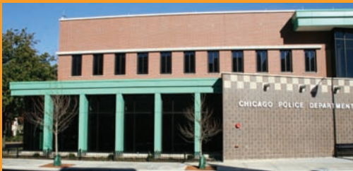
23rd District Police Station, Chicago (Source: Public Building Commission of Chicago)
