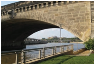
JFK Bridge over the Schuylkill River
