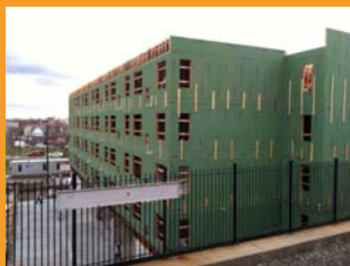
Paseo Verde - under construction
