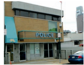
9th Police District Building on 21st Street
