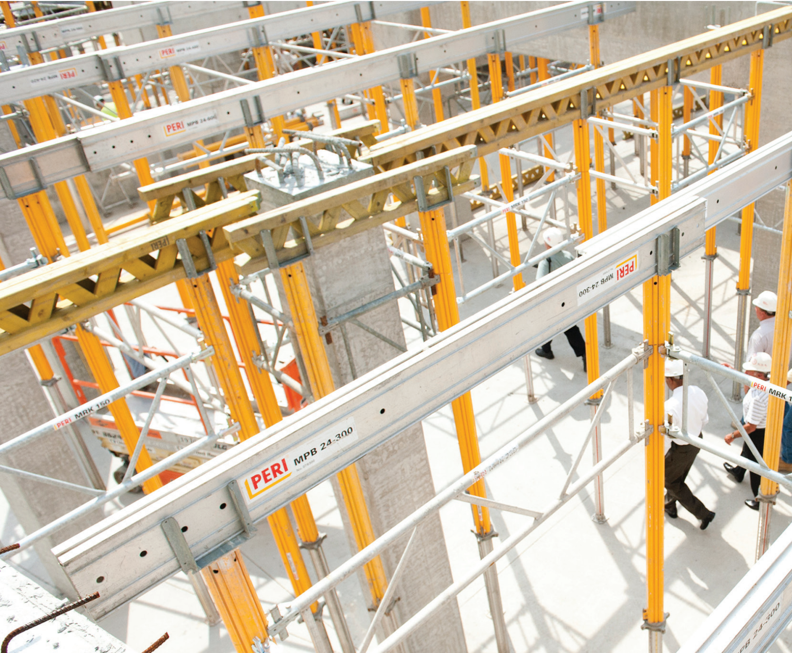
Construction in the Central District (Source: Kait Privitera)
