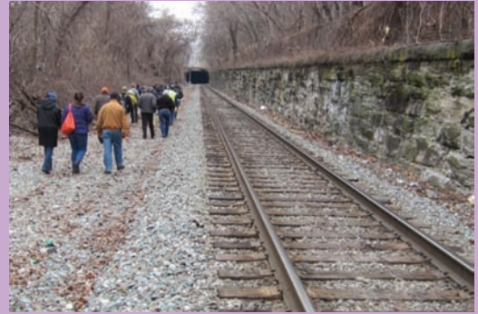
City Branch rail cut
