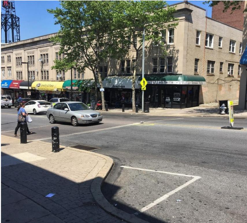
Figure 17: Mid-block crossing on 69th Street with bump-out, signage, and clearly marked crosswalk.
