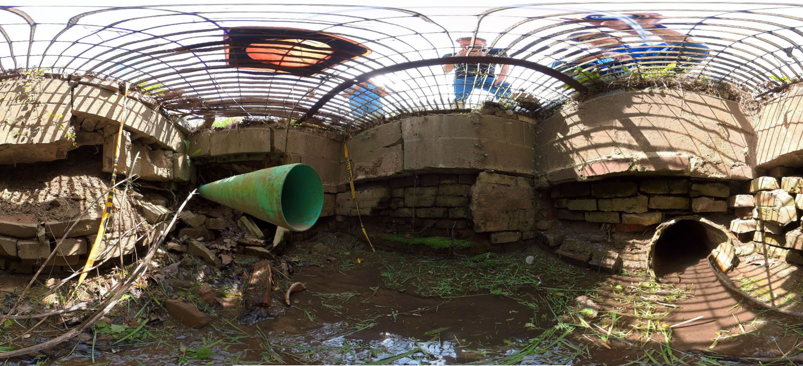
Using Insta360 Camera for Inlet Inspection
