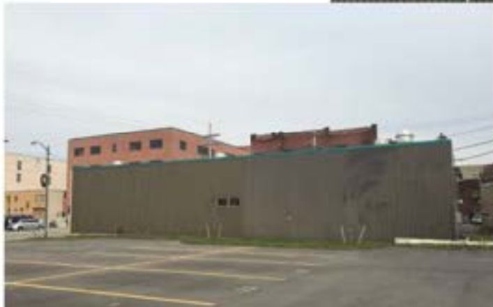
The Meadville Club prior to demolition
