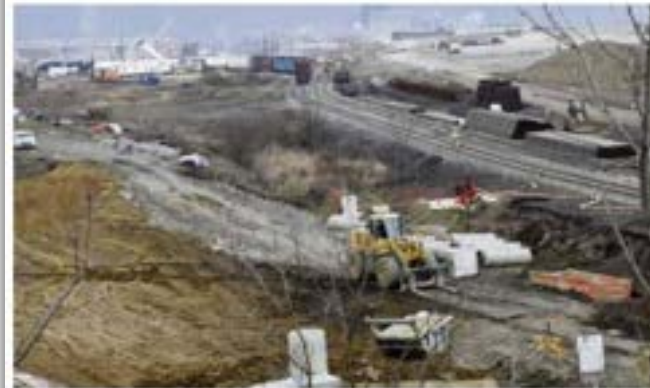
Site preparation and road work continue Friday, Dec. 11, 2015, along Route 18 in Beaver County at the site of Shell's planned ethane cracker.
