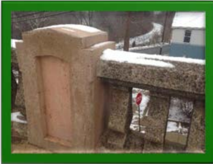
Schuylkill Avenue Bridge, Reading
