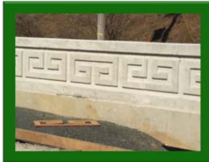
Buttonwood Street Bridge reconstructed parapets
