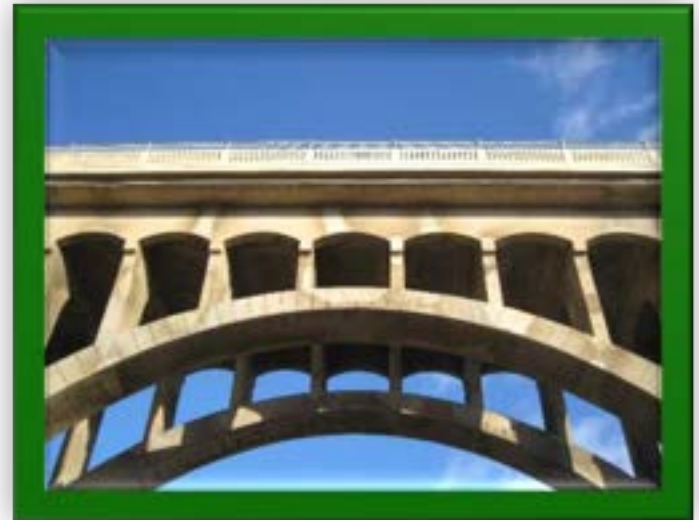
8 th Street Bridge, Allentown
