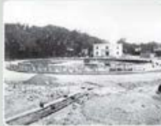
Construction of Bartholdi Park 1932
