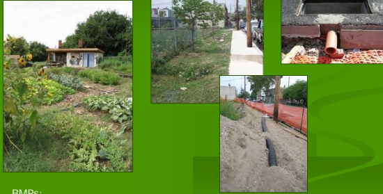
BMPs: Inlet Disconnection; Vegetated Swales; Green Roof
