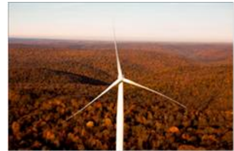
Mehoopany Wind Farm – Wyoming County
