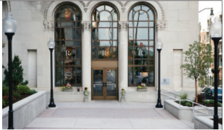
RENAISSANCE HOTEL EXTERIOR
