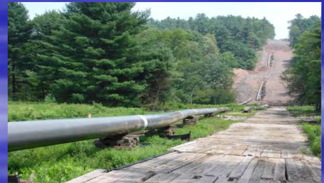
Gas Line Installation
