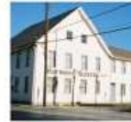
Village Center in Harmony, Pennsylvania
