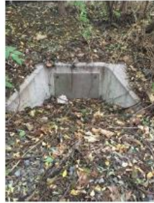
Picture 4 - Outlet pipe completely blocked with sediment, silt, and debris.
