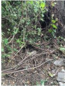
Picture 1 - Overgrown vegetation observed throughout detention basin.
