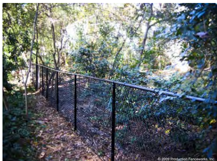
Image 39 Typical 8' Vinyl Coated Chain Link Safety Fence
