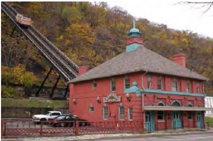
Image 10 The Monongahela Incline at East Carson Street.
