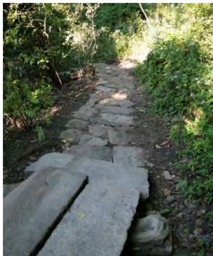
Image 18 A stone drainage crossing and paved trail built by the SCA in the Mount Washington Park area.
