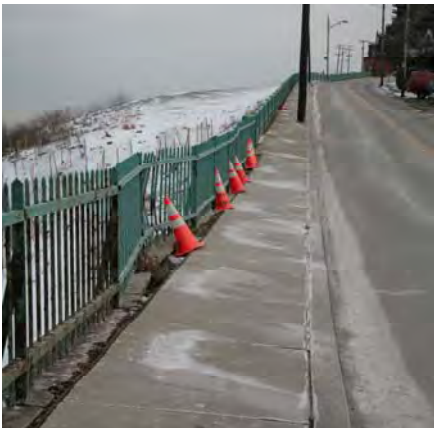
Image 11 Sidewalk and railing condition along Grandview Avenue at the terminus of Shaler Street.
