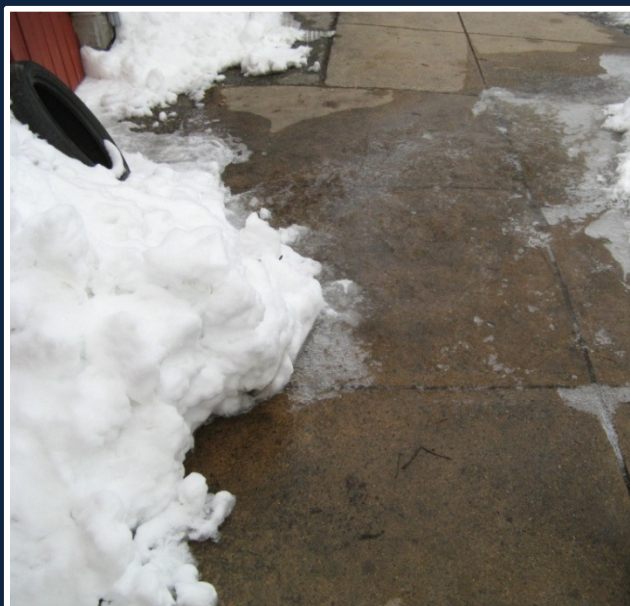
Ice formation due to down spouting and refreezing of melted snow
