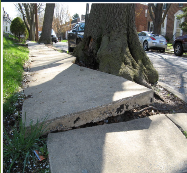
A sidewalk uplifted by tree roots on Madison Street
