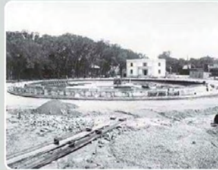
Construction of Bartholdi Park 1932
