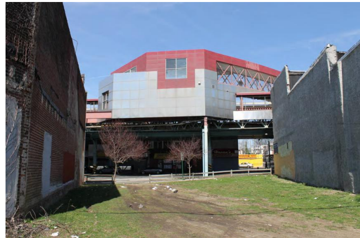
view from the sidewalk
