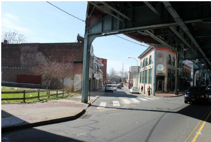
view of Frankford Ave from the site
