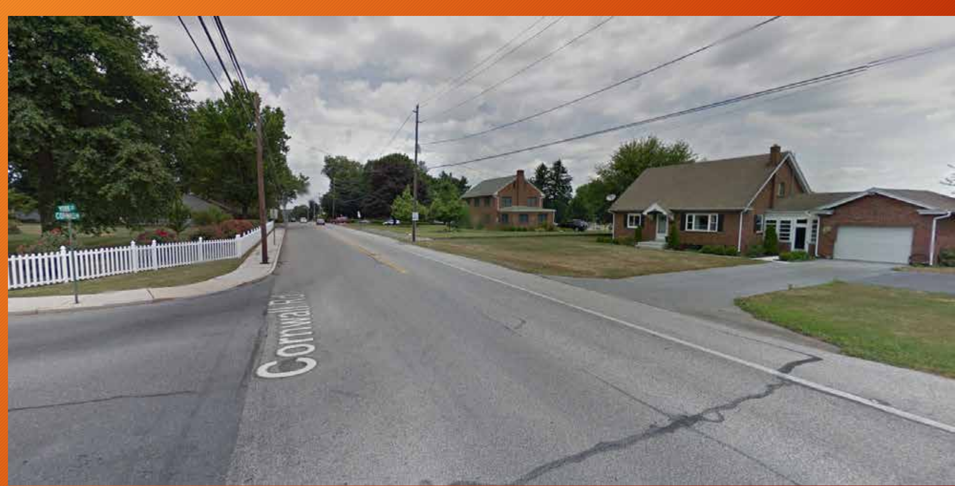
Cornwall Road (SR 2001) and York Street intersection looking North
