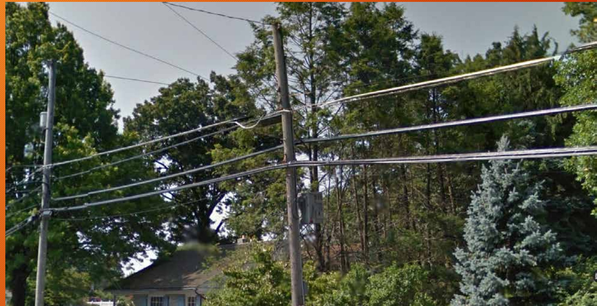
View of public utilities junction box at northeast corner of Wilhelm Ave and Cornwall Road Intersection
