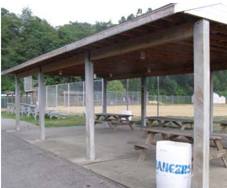
The existing pavilion is in good condition and should remain.
