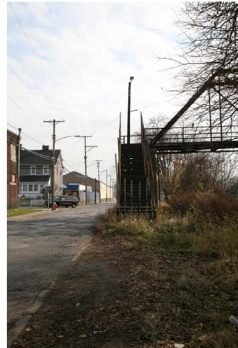
The Presston Bridge formerly connected Island Avenue to the Presston neighborhood and is planned for demolition. Residents have asked that pedestrian access to Island Avenue be re-established via a new bridge connector.
