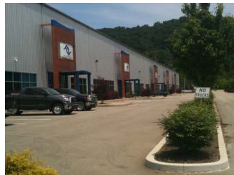
An example of a flex-office development situated in Leetsdale, PA.
