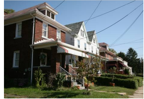
Example of a stable residential neighborhood with McKees Rocks.
