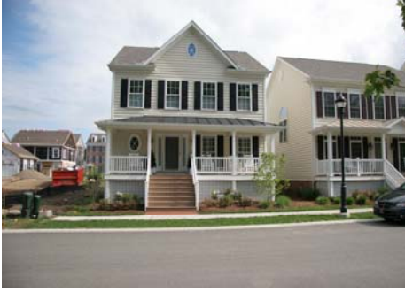
An example of constructing a residential neighborhood within a flood plain can be found in Chapel Harbor on the Allegheny River.
