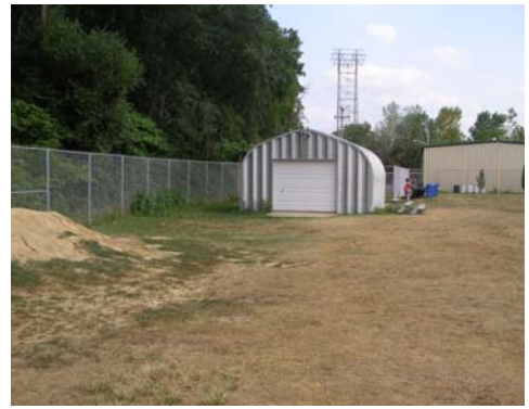
The maintenance building could benefit from landscape screening and improved equipment access.
