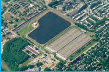
Queen Lane Reservoir (Source: 2010 Pictometry International Corporation Rochester, NY)
