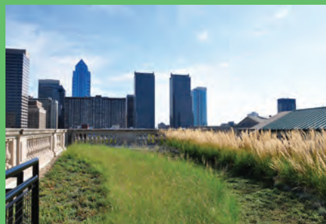
The main branch of the Free Library's planted roof. (Source: Mayor's Office of Sustainability)
