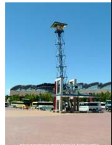
Photovoltaic Towers in Olympic Park, Sydney
