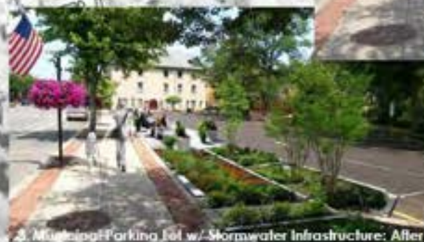
3. Municipal Parking Lot w/ Stormwater Infrastructure: After
