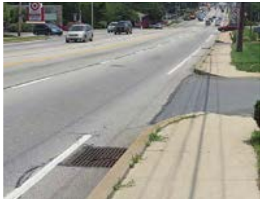
Stormwater grate at Travelodge entrance
