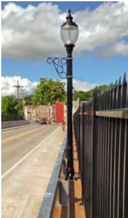
Pedestrian pole with globe fixture
