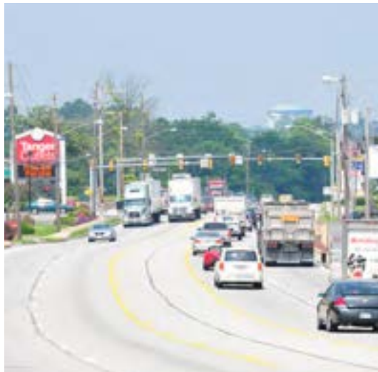
Typical roadway section with center turn lane
