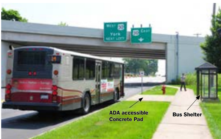
Example of enhanced bus stop detail
