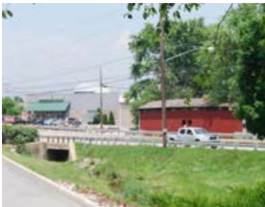
Drainage area at Rockvale Outlets
