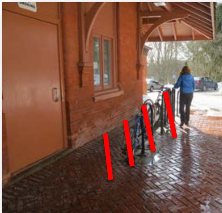
Rosemont Station – Paoli Thorndale Line
