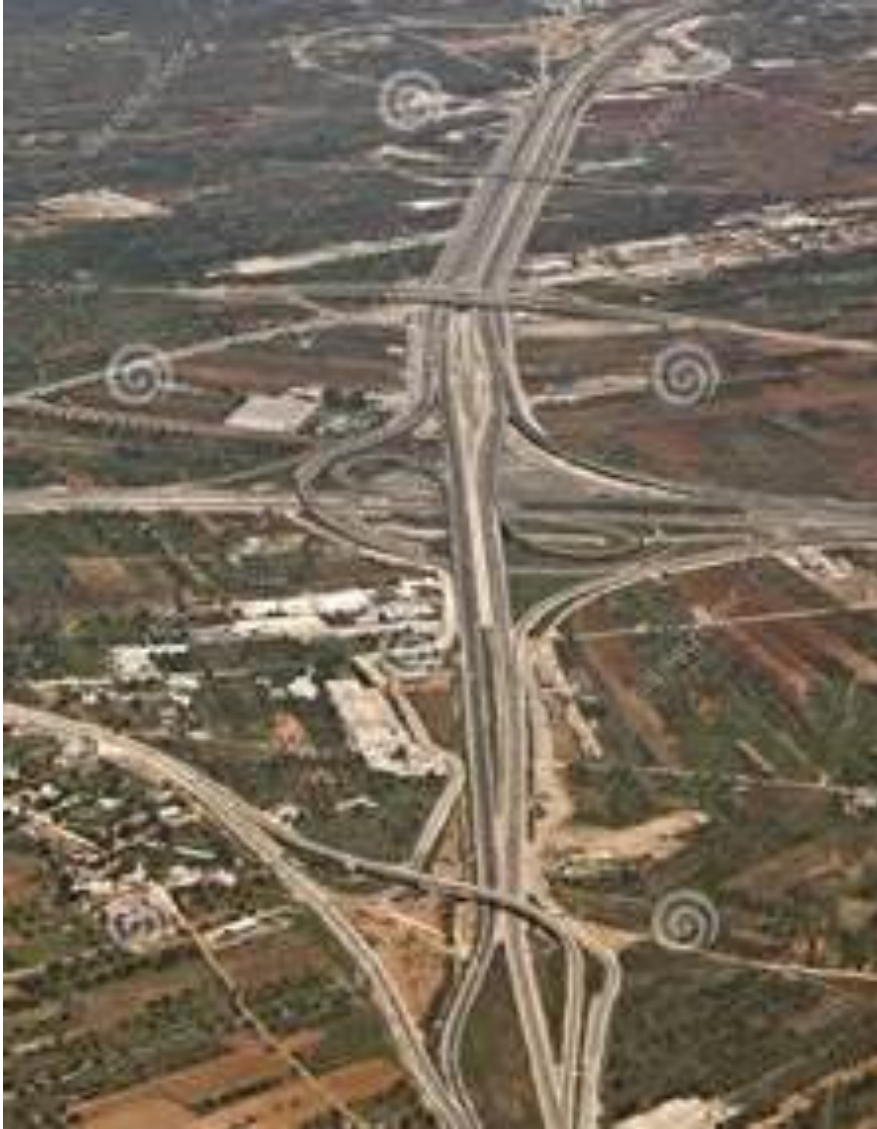
Linear Highway Infrastructure
