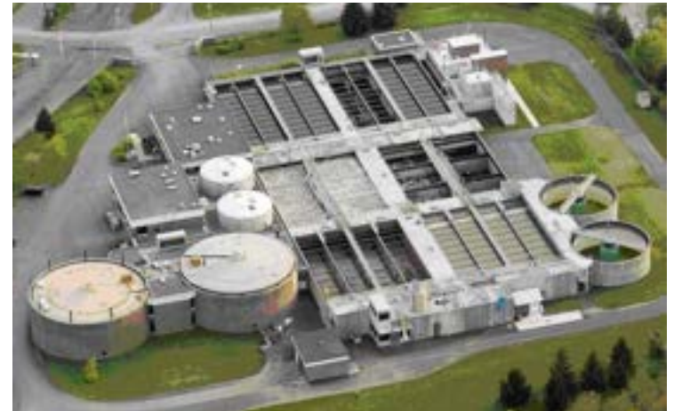
Conventional Sewer Plant
