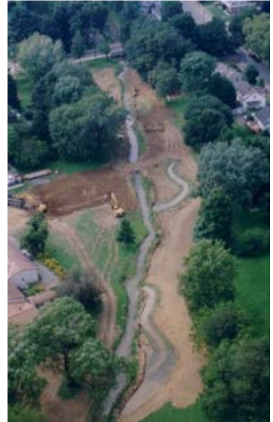
New Street Park floodplain restoration (during construction, 2005)
